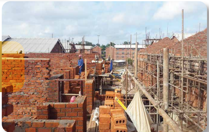
Adbenie Flats -Hualong Construction
